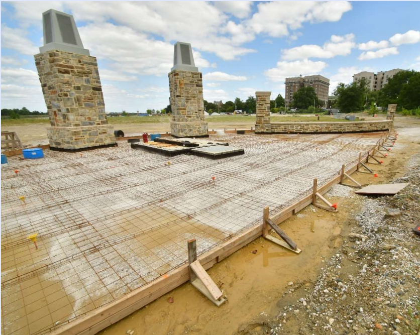
Tank 2 Access Area – 8/20/2024
