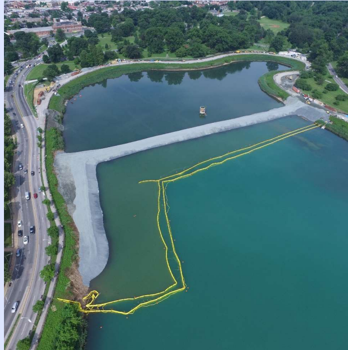
Cofferdam & Turbidity Curtain Completed - 6/8/2018
